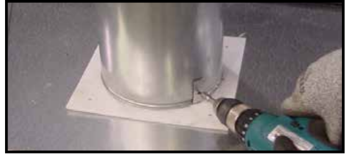
Figure 9.3 Gasket in Place
