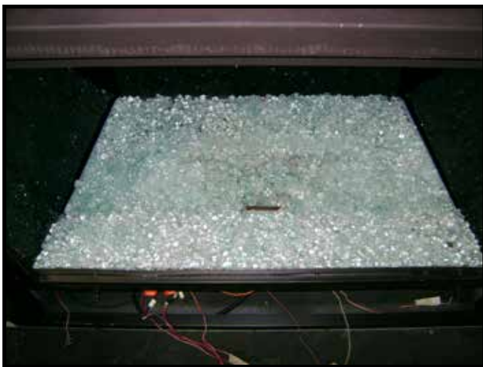
Figure 14.9 Proper Placement of Media
