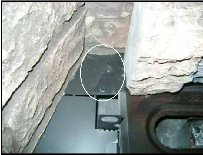
Figure 3.7 Remove Screws from Log Tabs
