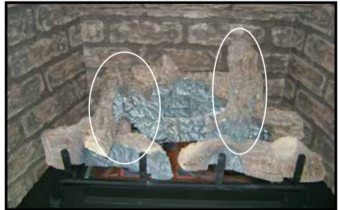
Figure 3.5 Remove Top Two Logs
