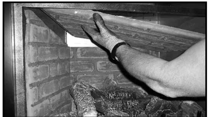
Figure 7.10 Remove Top Refractory
