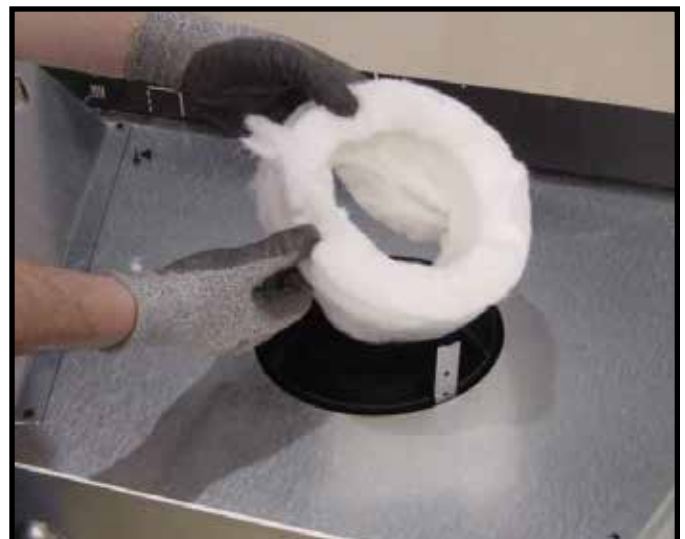
Figure 9.5 Remove the insulation from the outer vent pipe. For rear venting there is no insulation in the outer vent pipe.
