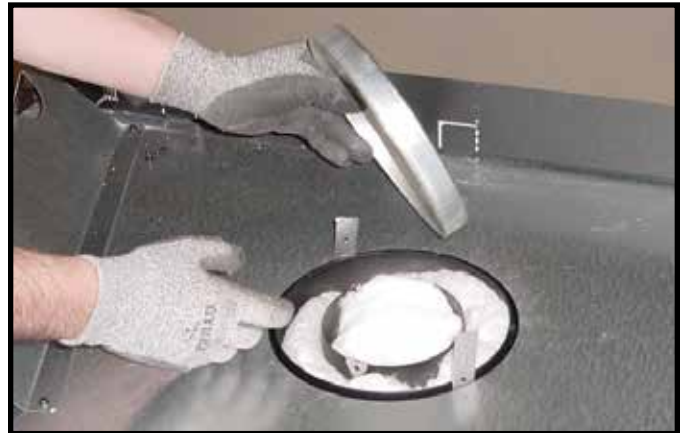
Figure 9.3 Remove the seal cap.
