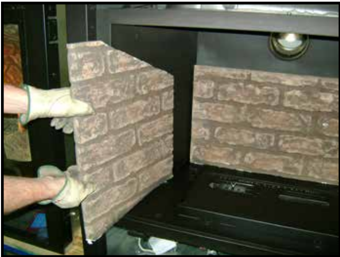
Figure 3.3 Side Refractory Removal
