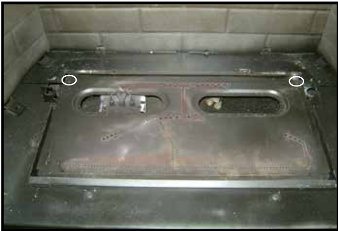
Figure 3.8 Remove Screws from Burner Assembly Rear Corners
