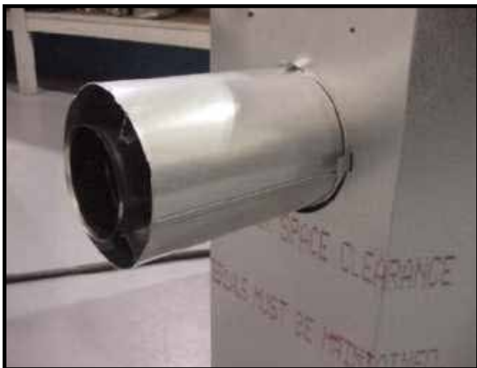
Figure 9.11 Attach the first vent section (it will snap into place). Slide the insulation gasket onto the vent section, up against the appliance and over the tabs.
