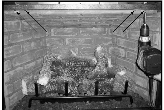
Figure 7.8 Remove Refractory Retainers
