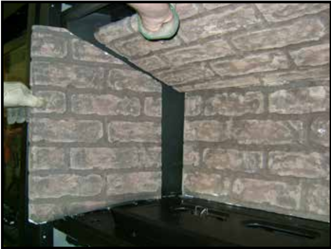
Figure 3.2 Top Refractory Removal
