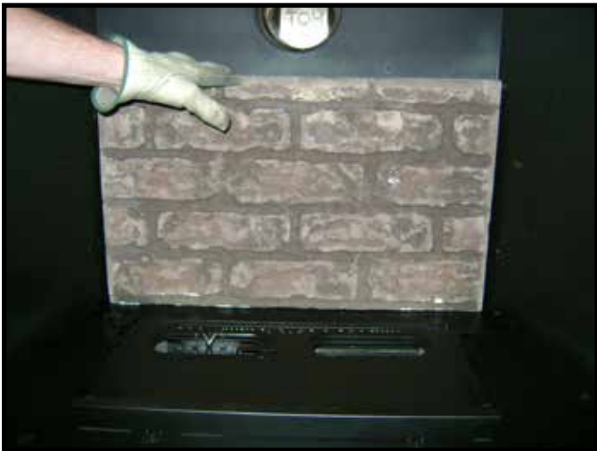
Figure 3.4 Back Refractory Removal
