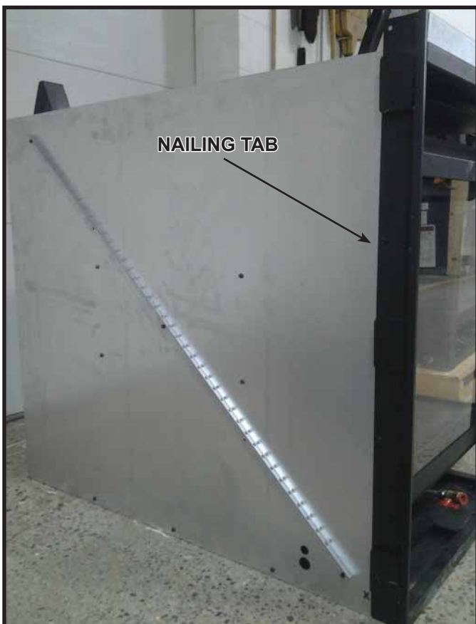
Figure 9.10 Attach Nailing Tab to Front Corner of Unit
