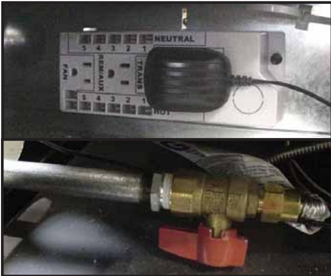
Figure 13.1 Preparation to Install Splatterguard
