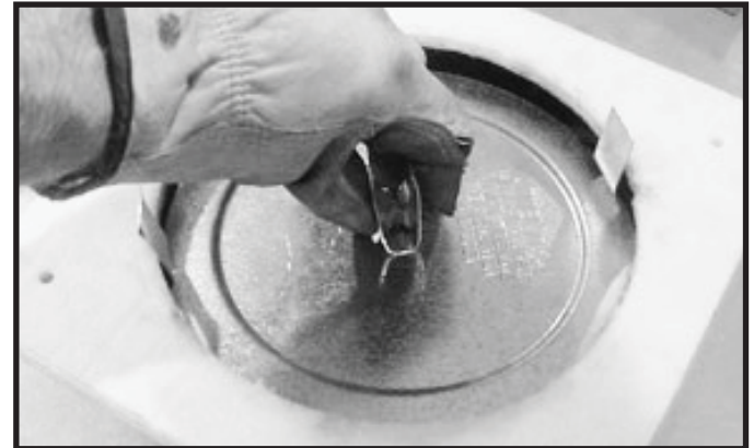
Figure 9.4 Fold the center parts of the retaining band up and use to remove the vent cap.
